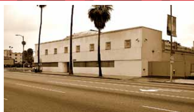
Western Recorders, 6000 Sunset Blvd, Hollywood, CA (Former location)
